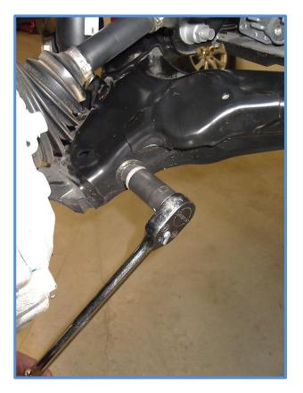
9. Once the factory shock has been taken off the vehicle, unbolt and remove the factory upper control arm by removing the long through bolt located behind the coil bucket. Install the King Coilover with the control arms removed then install aftermarket arms as per the instructions that came with your control arms.
